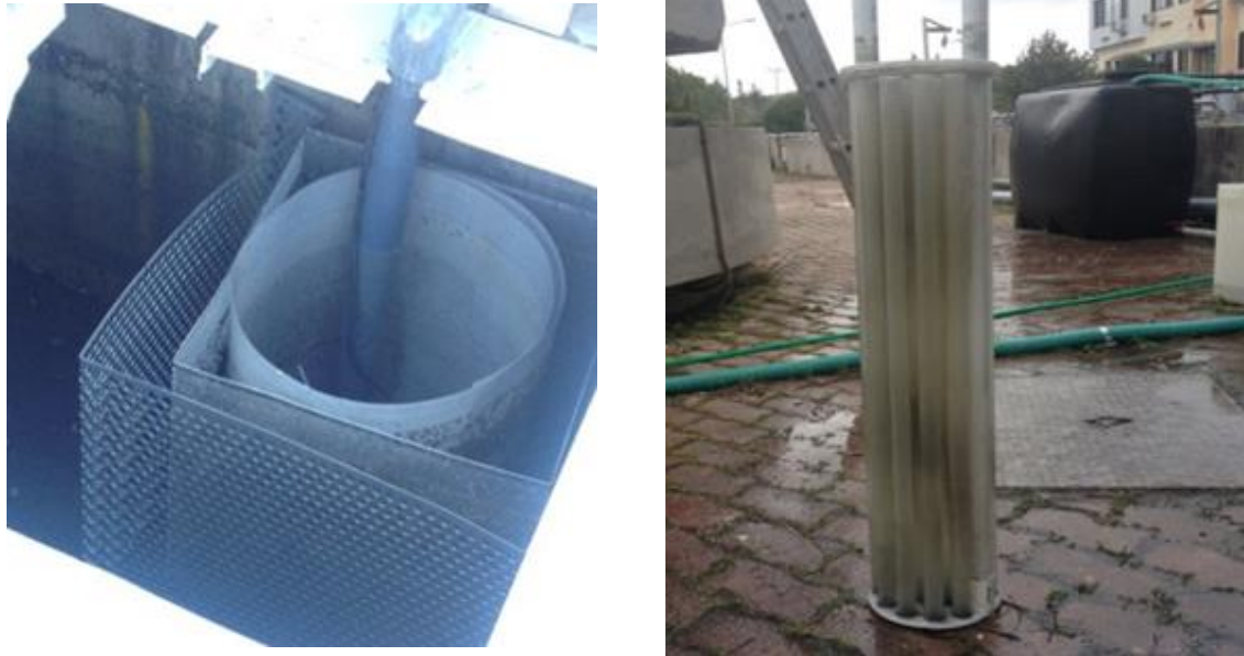
Figure 4. Presentation of the coarse screen ( \leq 5\text{mm} ) -grit system (left) and the biotube filter fine screen ( \leq 2\text{mm} ) (right) which constitutes the pretreatment stage.
