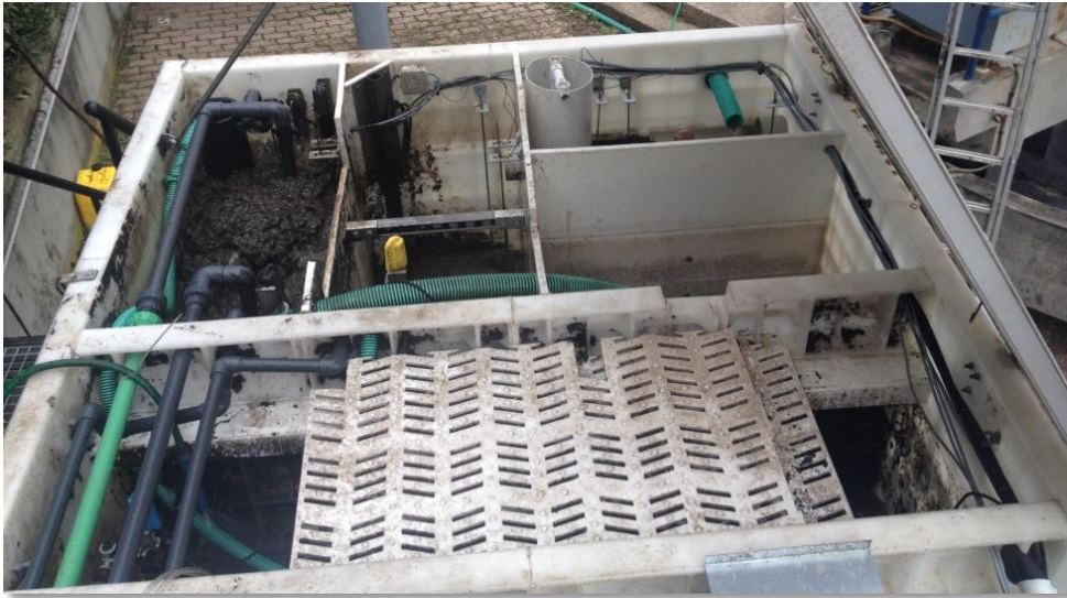
Figure 5. Presentation of the biological processing tank.
