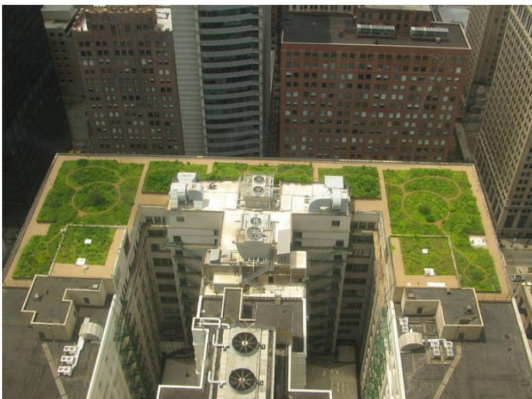
Figure 44. Example of green roof.
