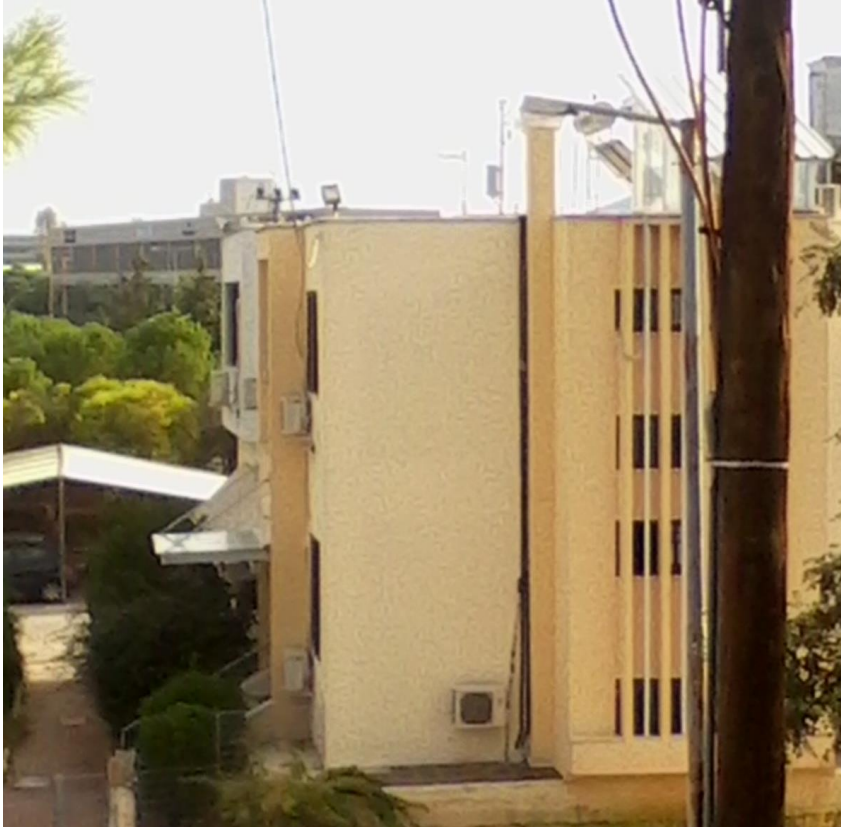
Figure 49. Multi-sensor on KEREFT building roof.
